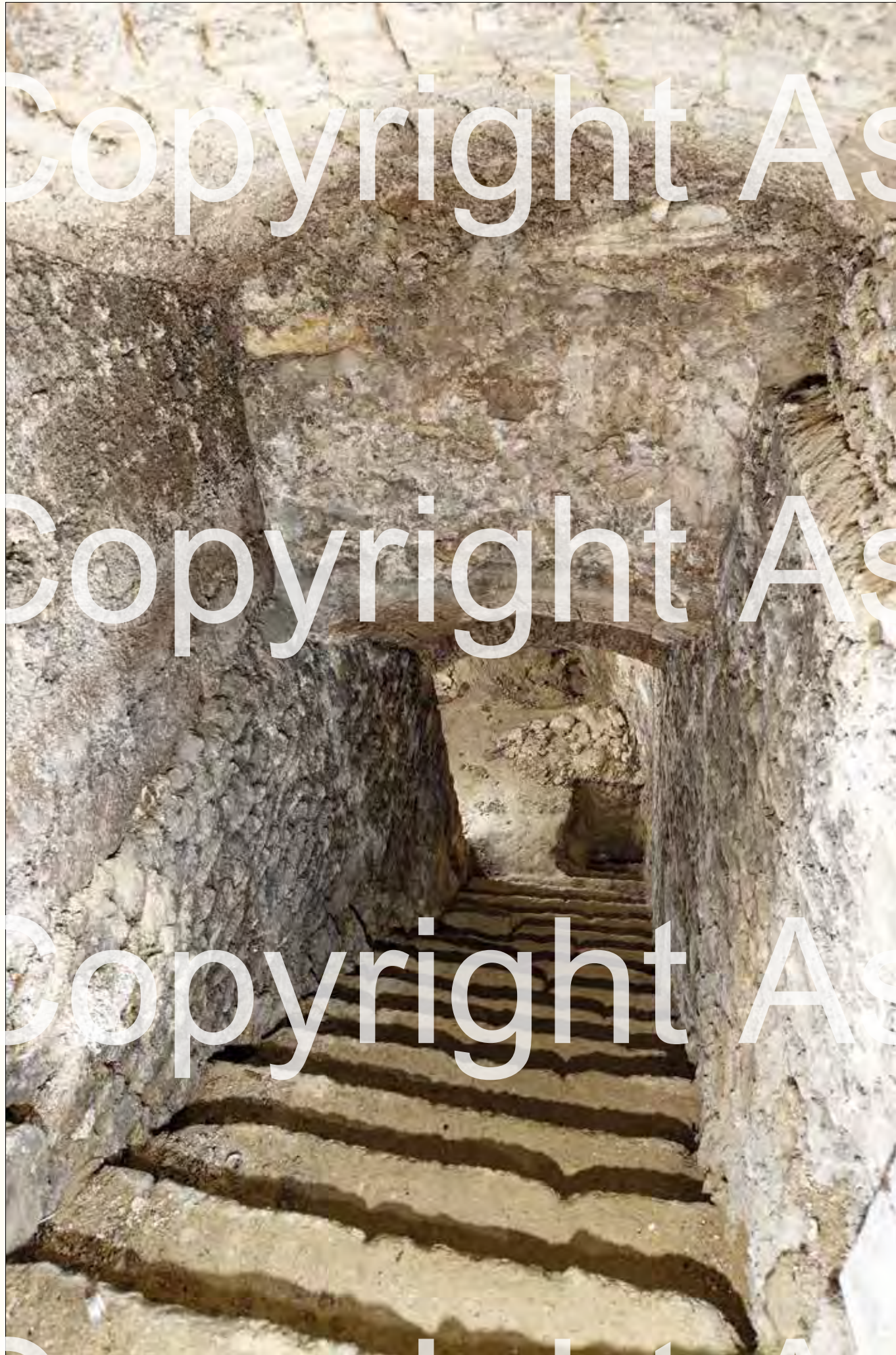
The vault of the staircase leading down into the quarry shows a slope break, probably before passing under the layer of non-friable stone.
