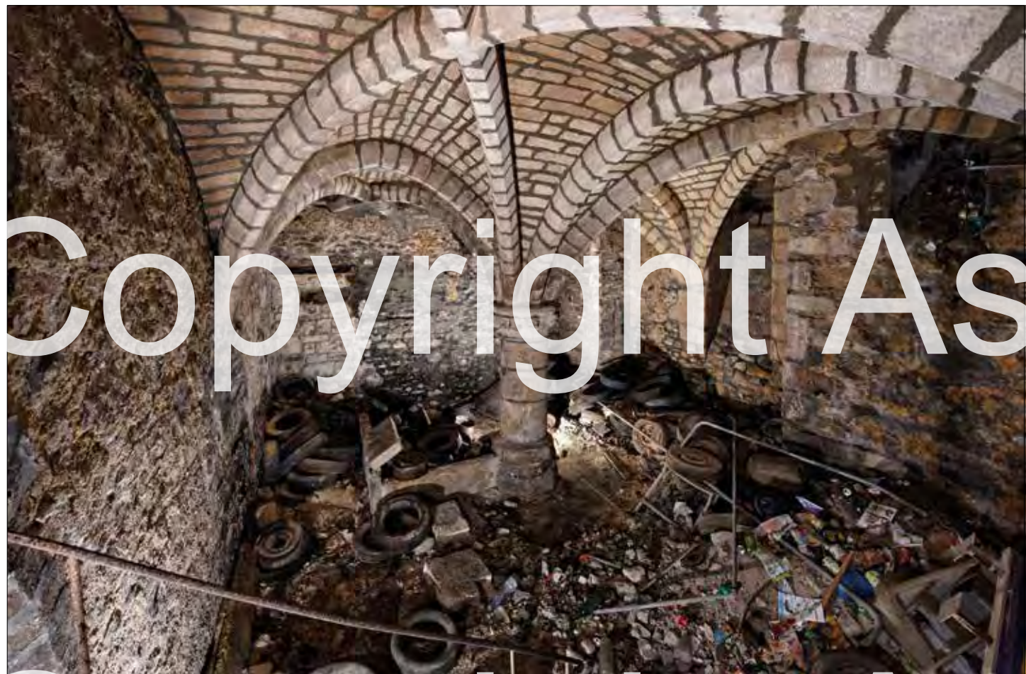
Very high 14th-century cellar, partially obstructed. The base of the arches merges into the walls.
