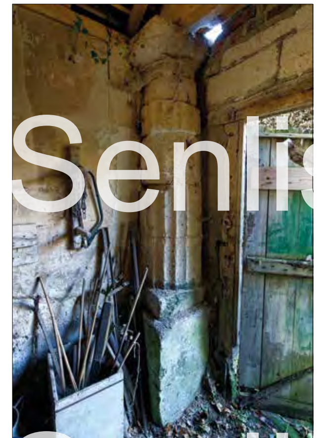
A support column in a small utility building, constructed from disparate elements.
