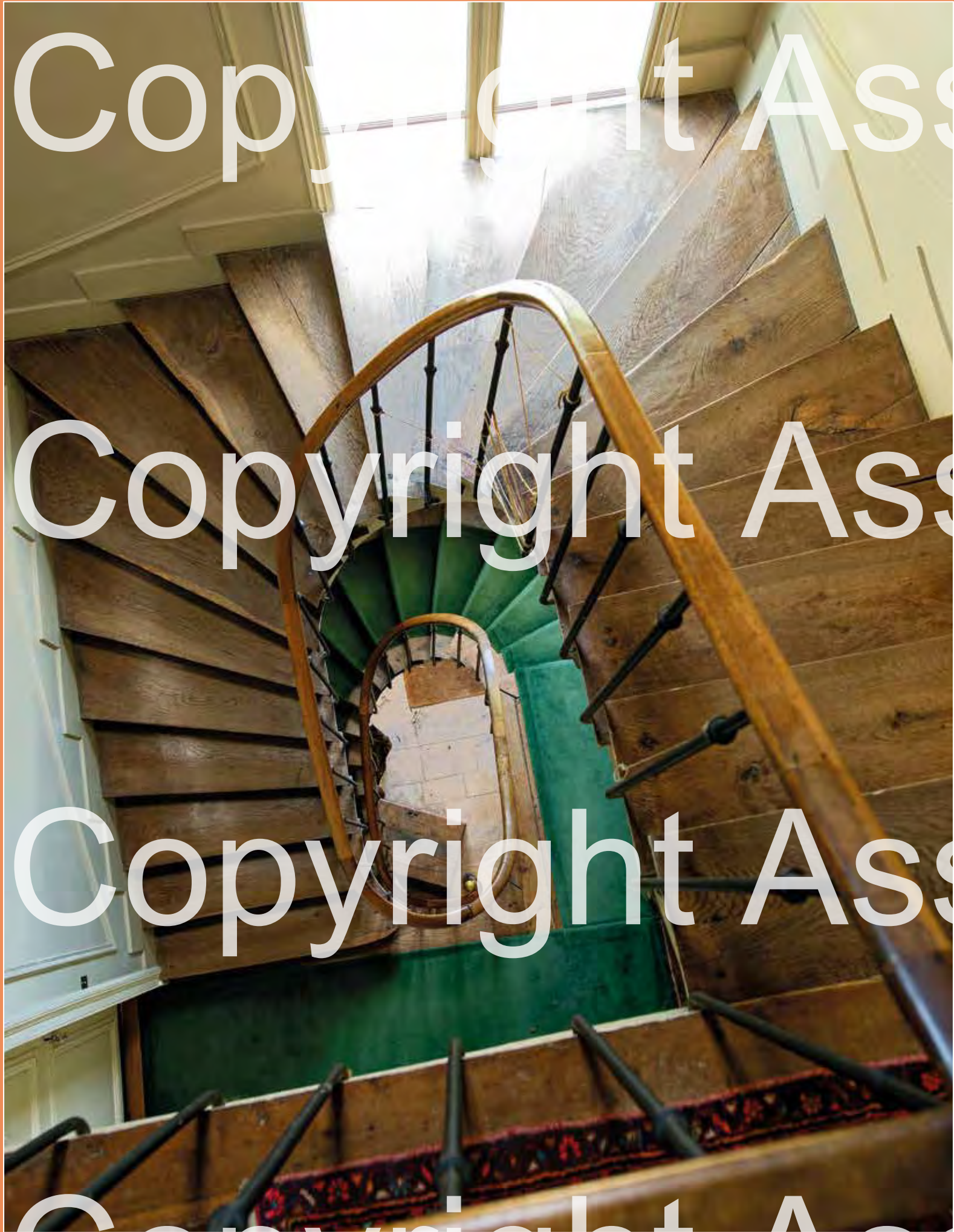
The wooden staircase is set within a square stairwell. However, most of the steps are winders, and the handrail is curved.
