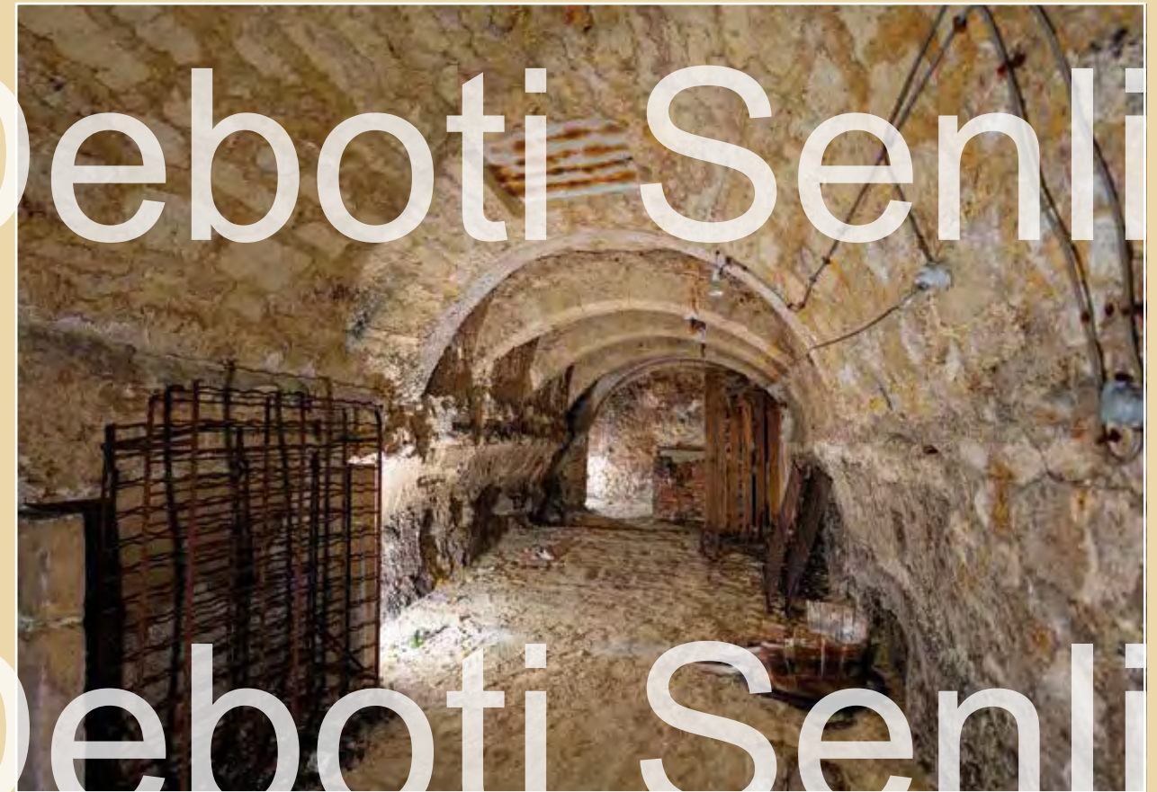
This corridor once connected two Gothic rooms at different levels. The deepest one is blocked off. The vault of the passage is made of masonry and reinforced at one end by four sturdy transverse arches. A ventilation duct has been blocked. The walls are cut from natural stone.
