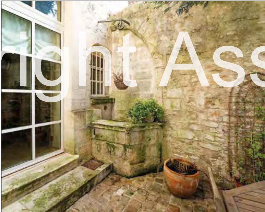
A shared well built into the party wall.
