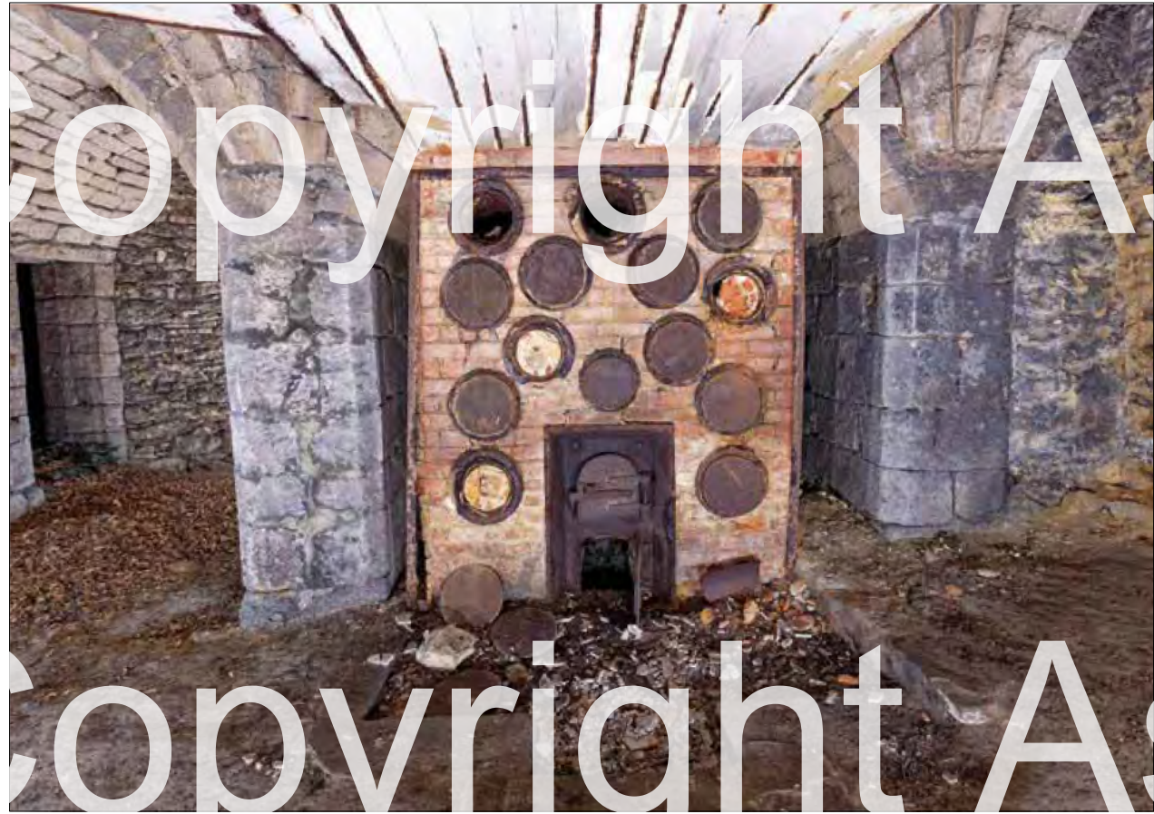
Such coal-fired central heating systems distributed hot air through a network of ducts and vents throughout the house. Installed in the 19th century, they took advantage of the vast cellars in Senlis. Most have been dismantled, like the one in the Musée de la Vénérice. This one, the best preserved, still has its ducts.
