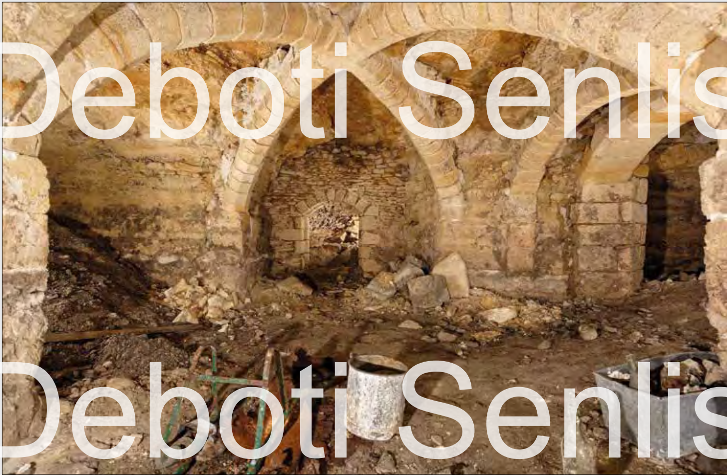
A crossroads of quarries reinforced with pointed arches.
