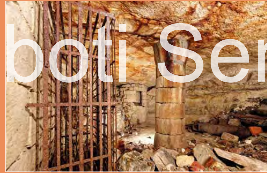
Each drum of this support column consists of two half-discs.
