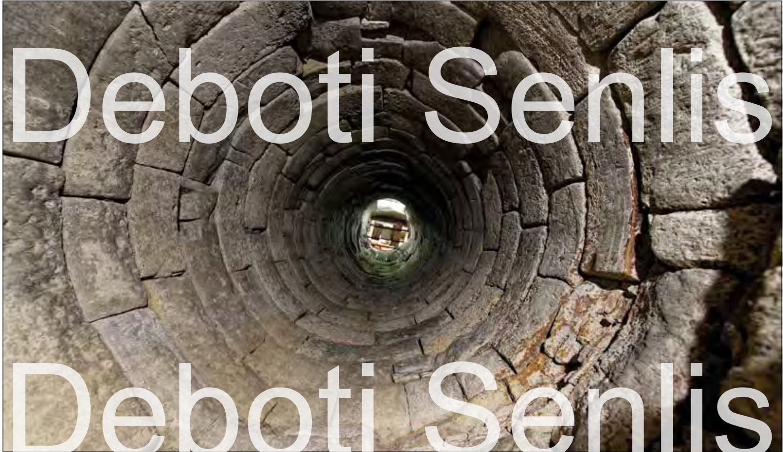
The view is taken from within the quarry; the shaft is entirely masonry-lined with carefully fitted stone. Daylight from the ground floor can be seen 12 metres above.
