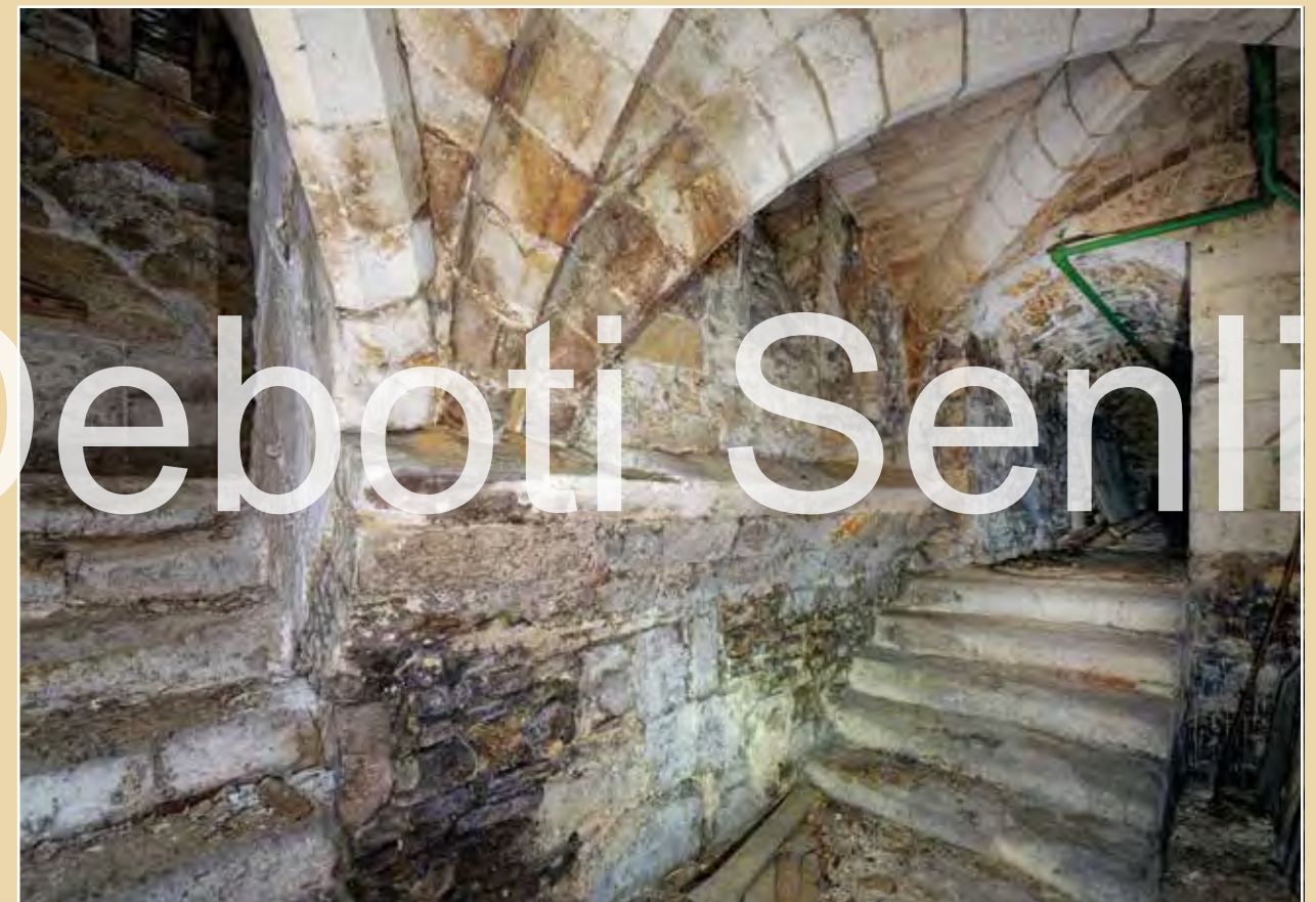
In this cellar, the remedial underpinning of the vault is clearly visible. Originally barrel-vaulted, it was later raised with ribbed vaulting.
