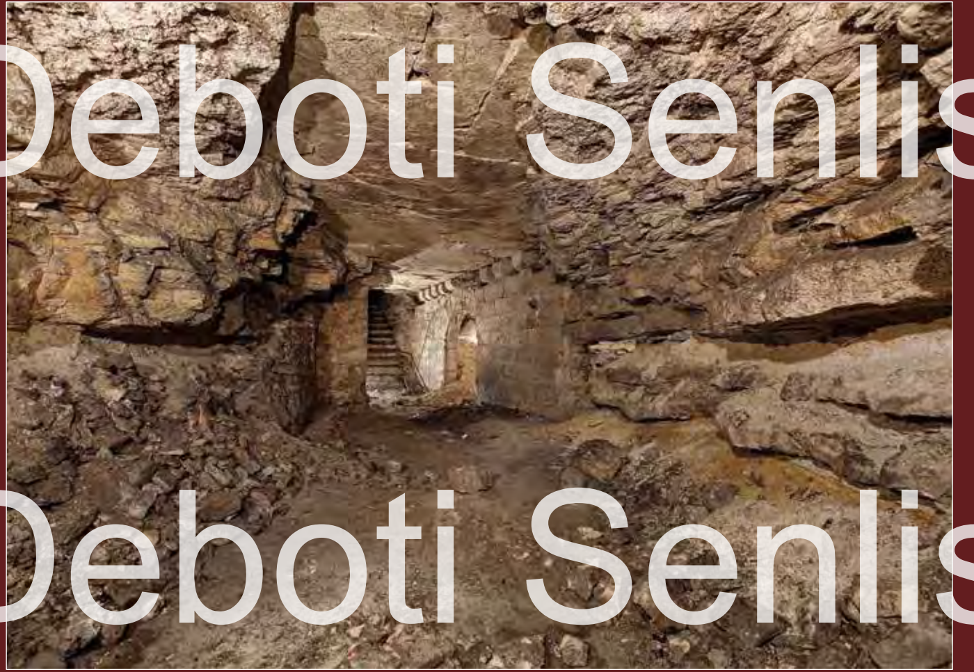
The quarry cellar beneath the storage cellar is divided by a wall constructed from reused stone.
