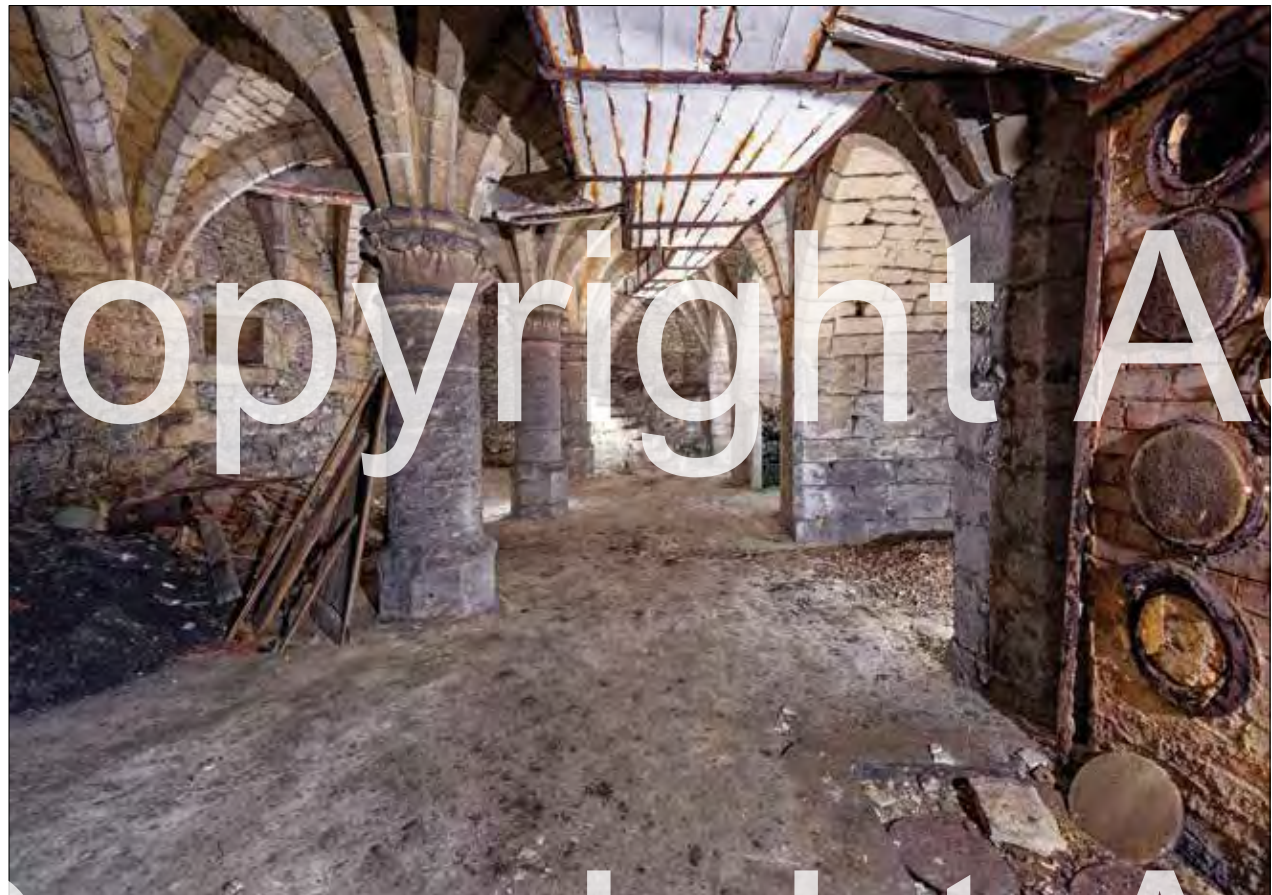
Such coal-fired central heating systems distributed hot air through a network of ducts and vents throughout the house. Installed in the 19th century, they took advantage of the vast cellars in Senlis. Most have been dismantled, like the one in the Musée de la Vénérice. This one, the best preserved, still has its ducts.
