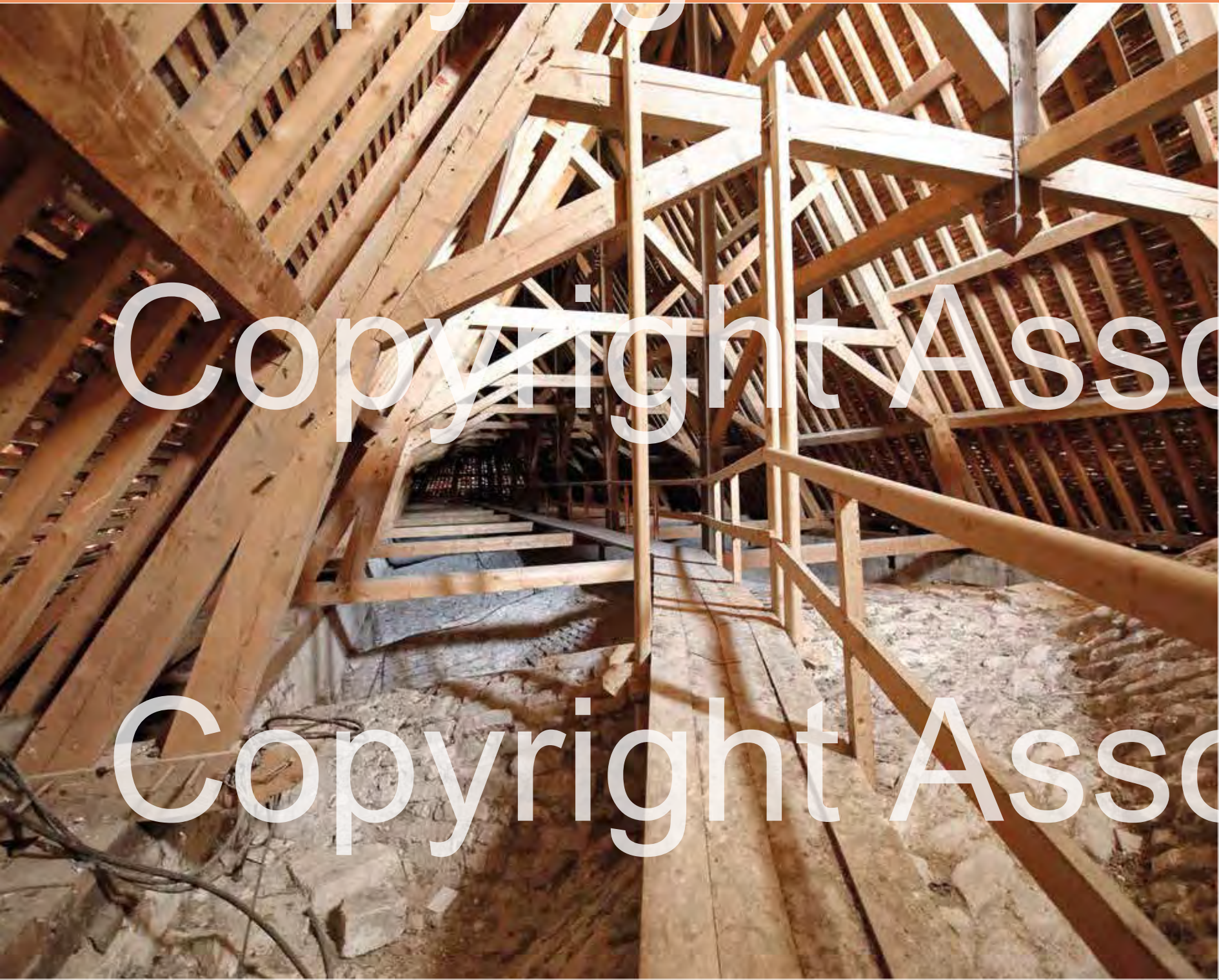
Modern roof structure (2004) over the vaults.
