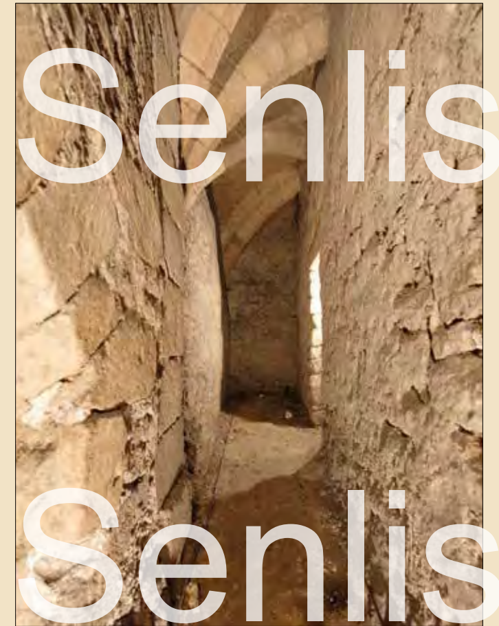
This narrow corridor is the result of underpinning a foundation wall beneath the lateral wall of the new house, which is narrower than the old one.
