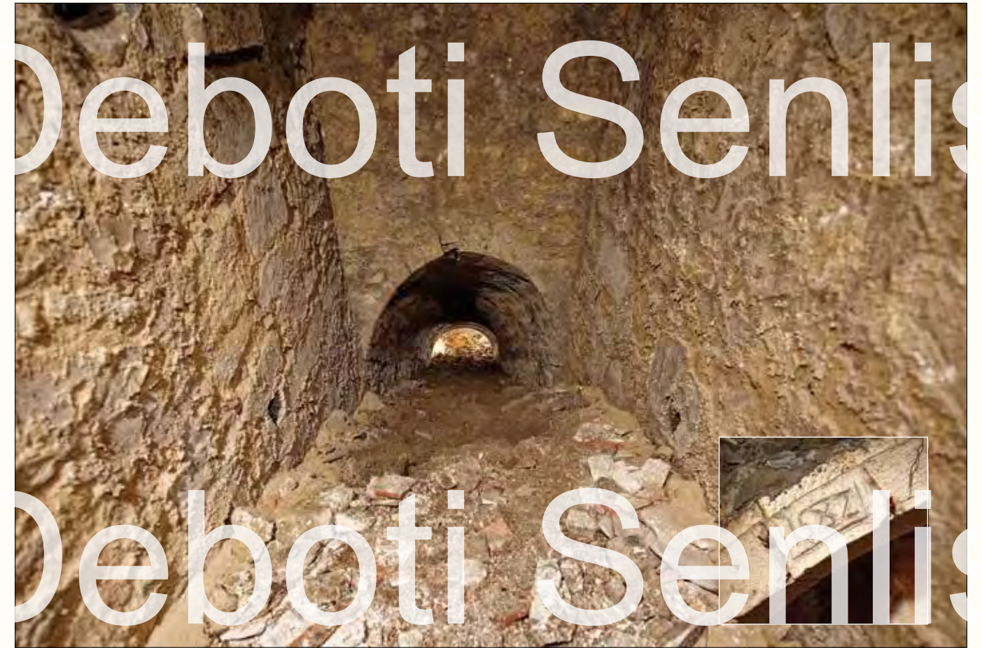
A vertiginous descent, largely filled in, that passes beneath the ancient rampart. The date '1582' at the start of the descent indicates that the vaulting was reconstructed at that point.
