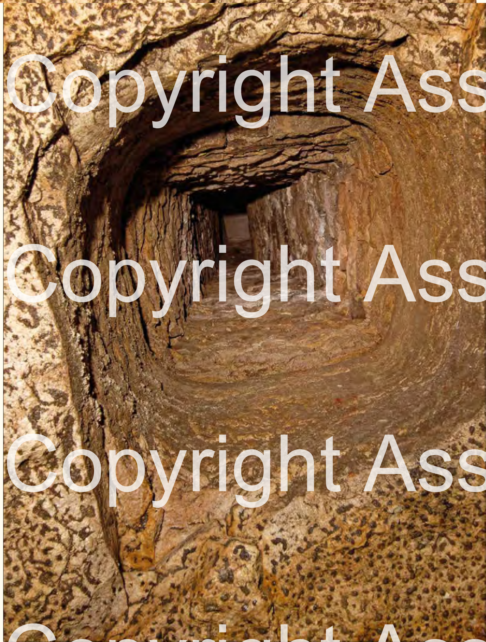
An extraction shaft in the quarry, 8 metres high.
