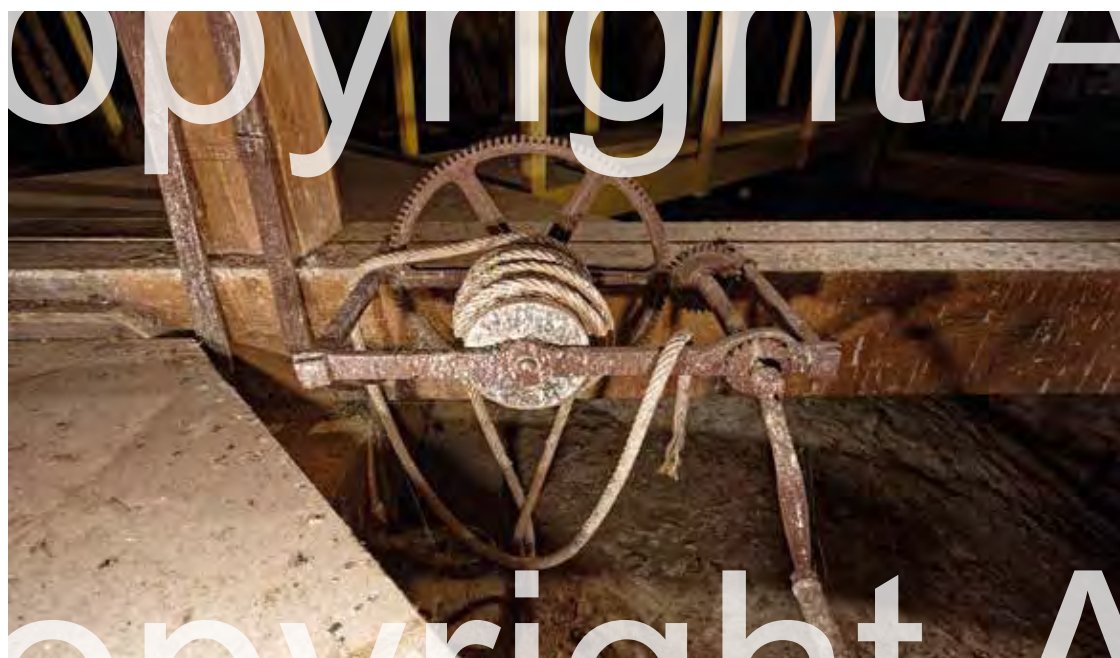
The pulleys and winches of the now disused light fittings remain in place.
