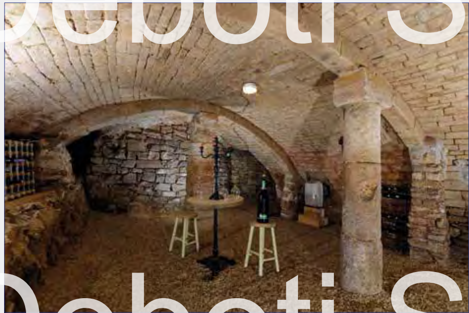
A wine-tasting cellar. Note the reinforcing columns to support the transverse arches.
