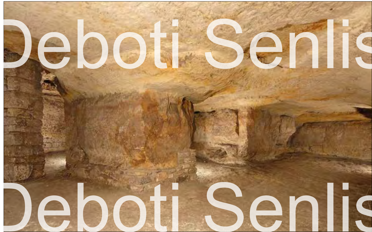
To the right, the quarry face clearly shows distinct marks from parallelepiped block extractions. In the center, the base of the natural pillar has been reinforced with masonry. To the left, a massive masonry pillar supports the ceiling of the quarry.
