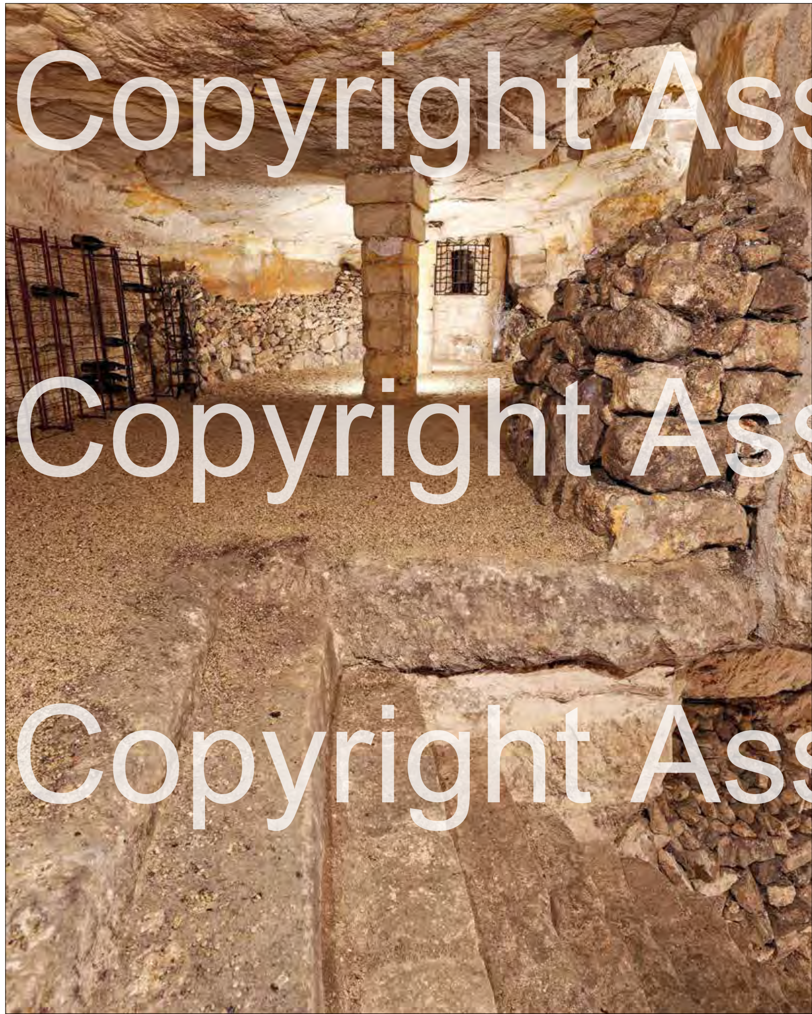
In this quarry cellar, various features can be found: at the back is the well; a quadrangular pillar supports the quarry; and loose, unmortared stones reinforce the base of the walls. In the foreground, a staircase descends to a second, deeper quarry.
