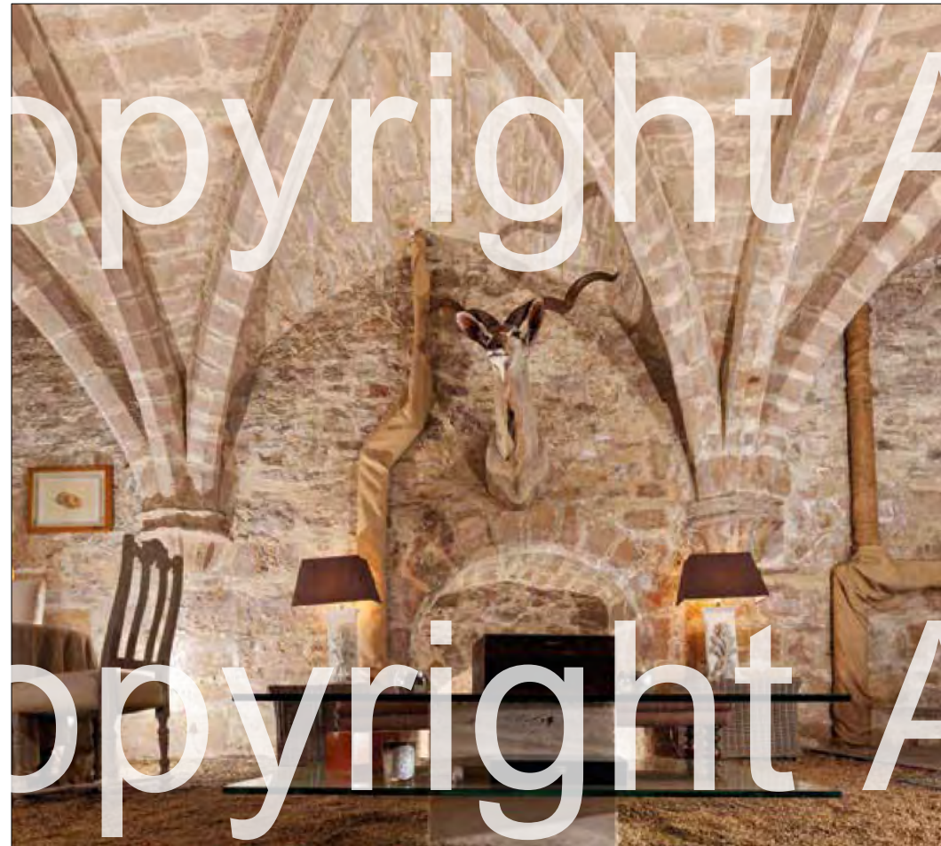
The springing of the arches on the walls is supported by corbels adorned with crockets.
