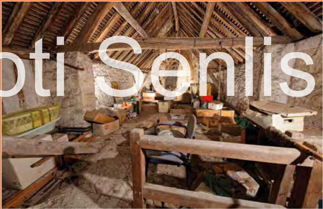
The tie-beam of the roof frame rests on the buttresses of the side walls, which may be remnants of an original gable before the house was extended.
