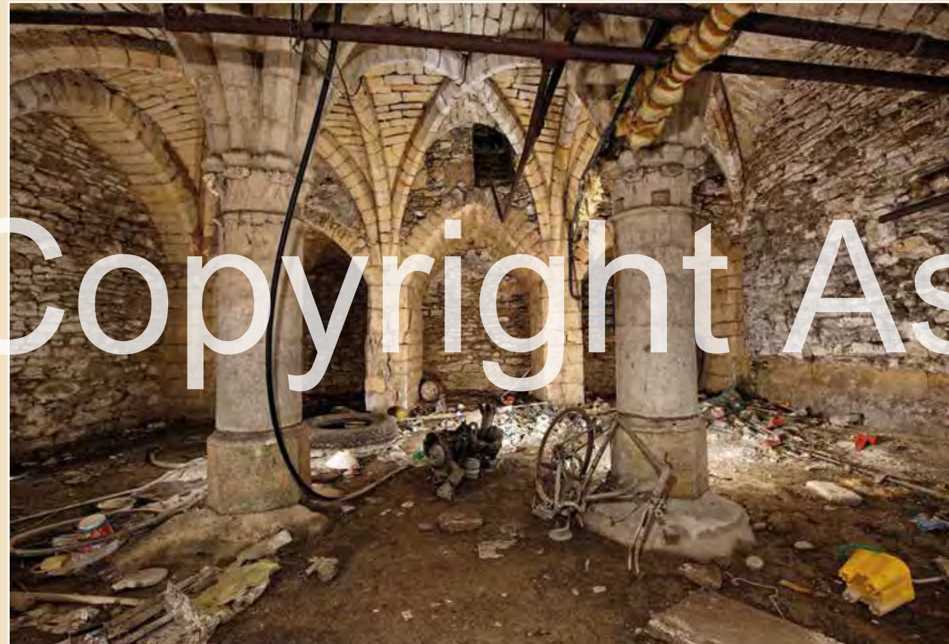
This may be the only Gothic cellar with four pillars defining three aisles and three bays. At the back of the room, monumental niches covered with pointed arches expand the usable space.
