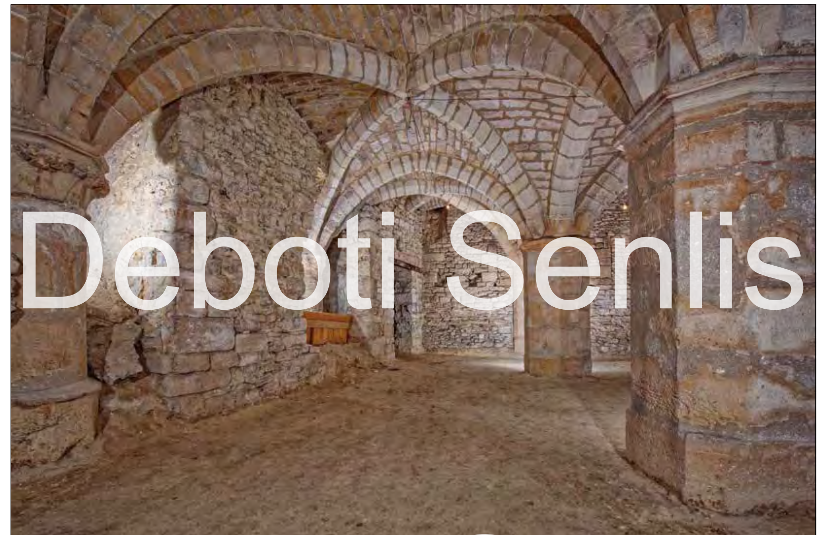
A cellar with a rib-vaulted ceiling. The arches rest on octagonal masonry columns in the middle of the room and on engaged columns along the walls, whose capitals feature crocket motifs.
