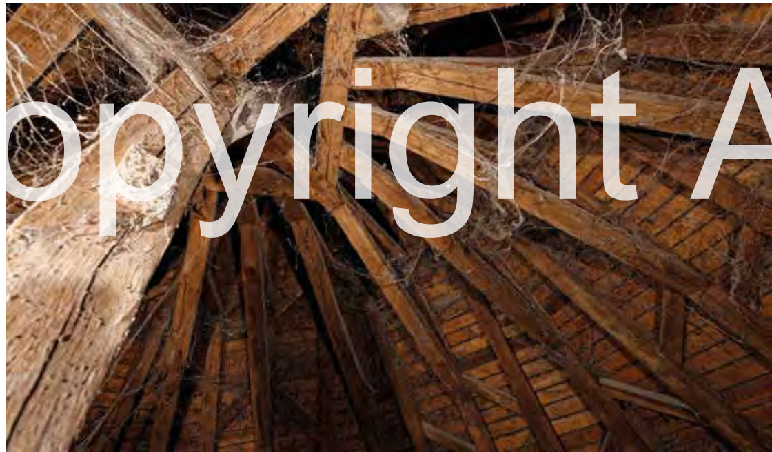
Structure of the apse roof frame: set of wooden pieces located on a horizontal plane and radiating around the post.
