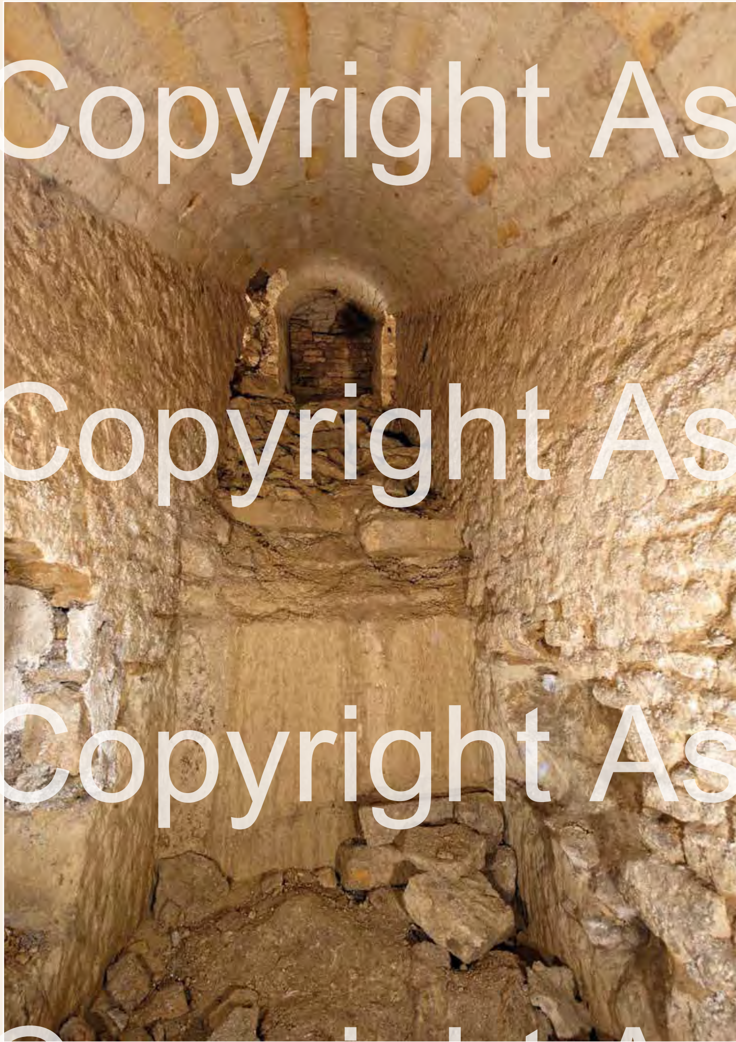
An abandoned quarry descent, formerly blocked. The staircase has been partly destroyed.
