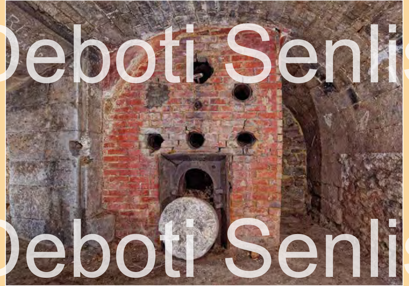
Another model of coal-fired heater installed in a barrel-vaulted cellar.
