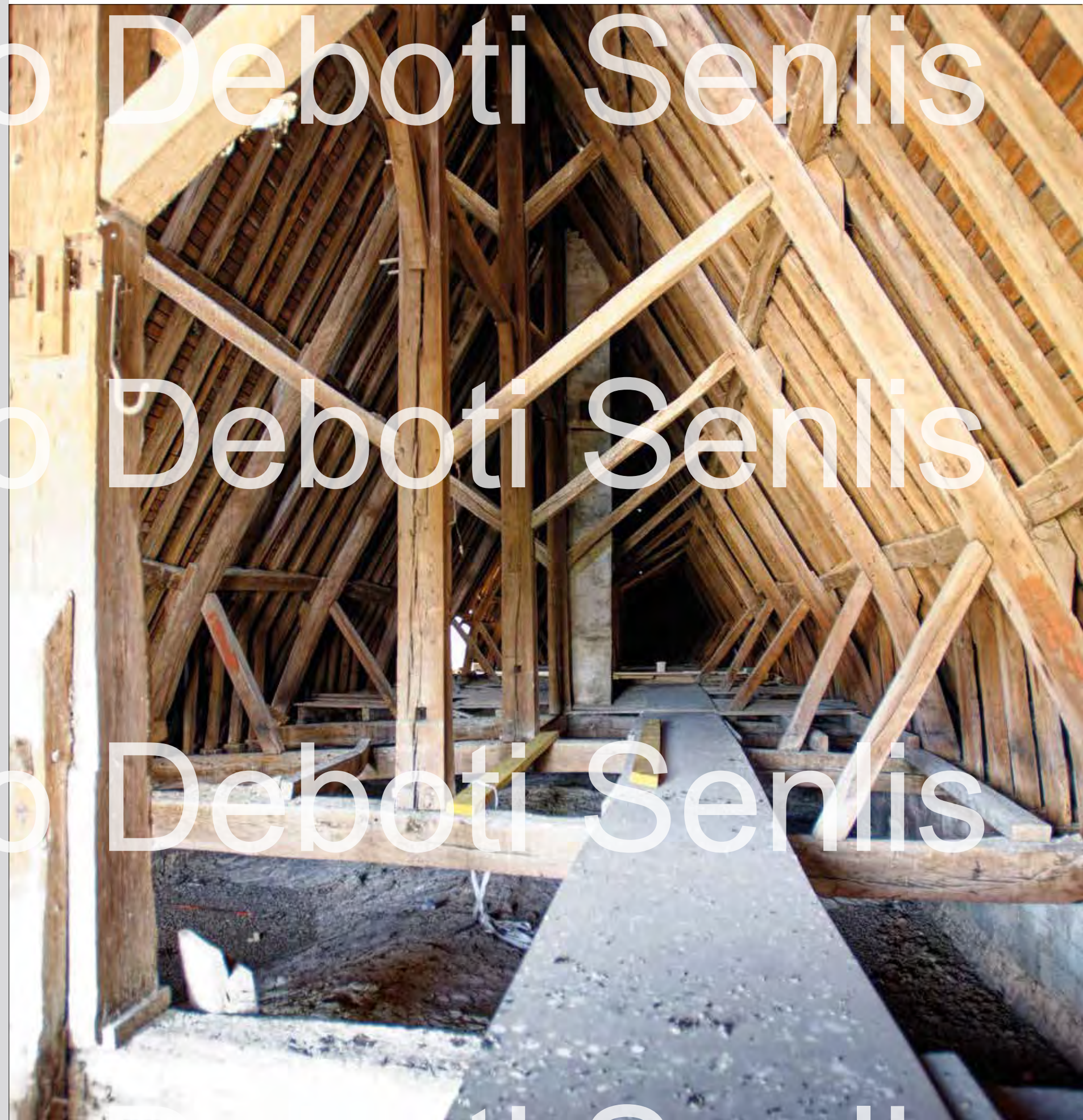
The steep slope of the roof explains the increased use of struts and bracing (oblique wooden pieces) on each truss of the framework.
