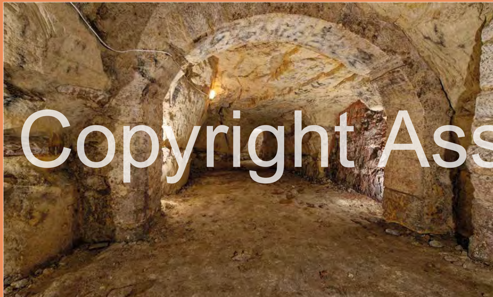
A quarry with a natural pillar supporting the ceiling.
