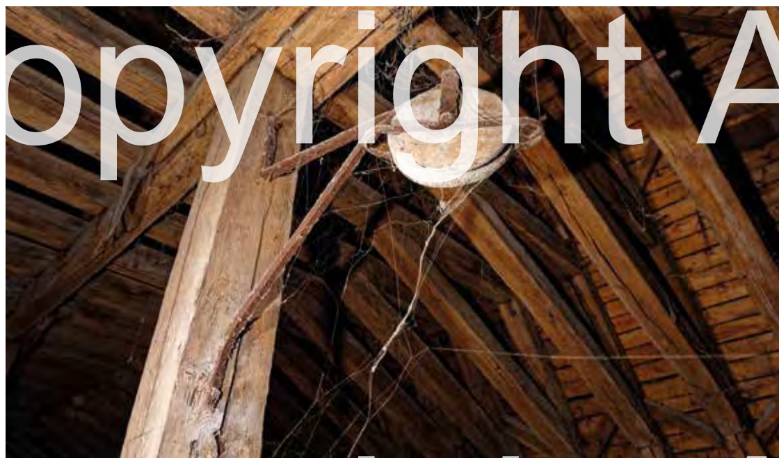
The pulleys and winches of the now disused light fittings remain in place.
