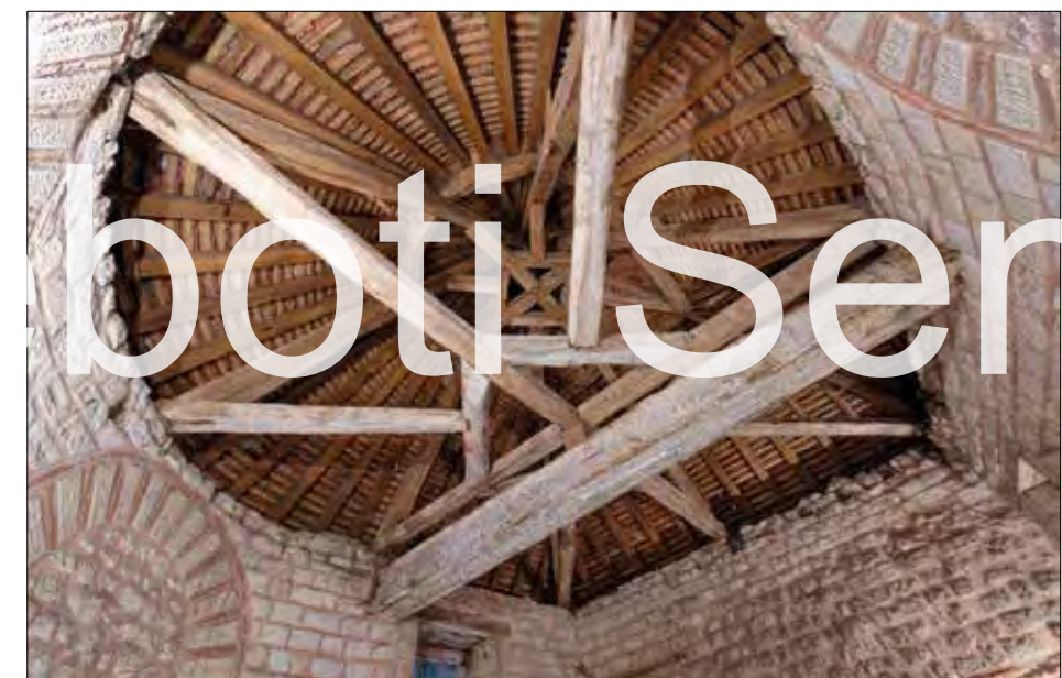
The wooden roof structure of the Gallo-Roman tower was spared in the bombardment.
