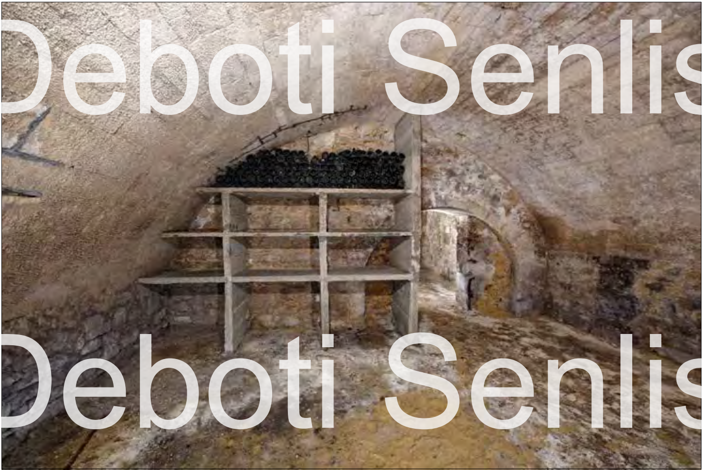
A barrel-vaulted cellar without pillars or transverse arches.
