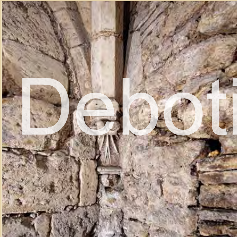
A cellar corner where arches rest on a capital adorned with crockets and a heavily damaged engaged column.
