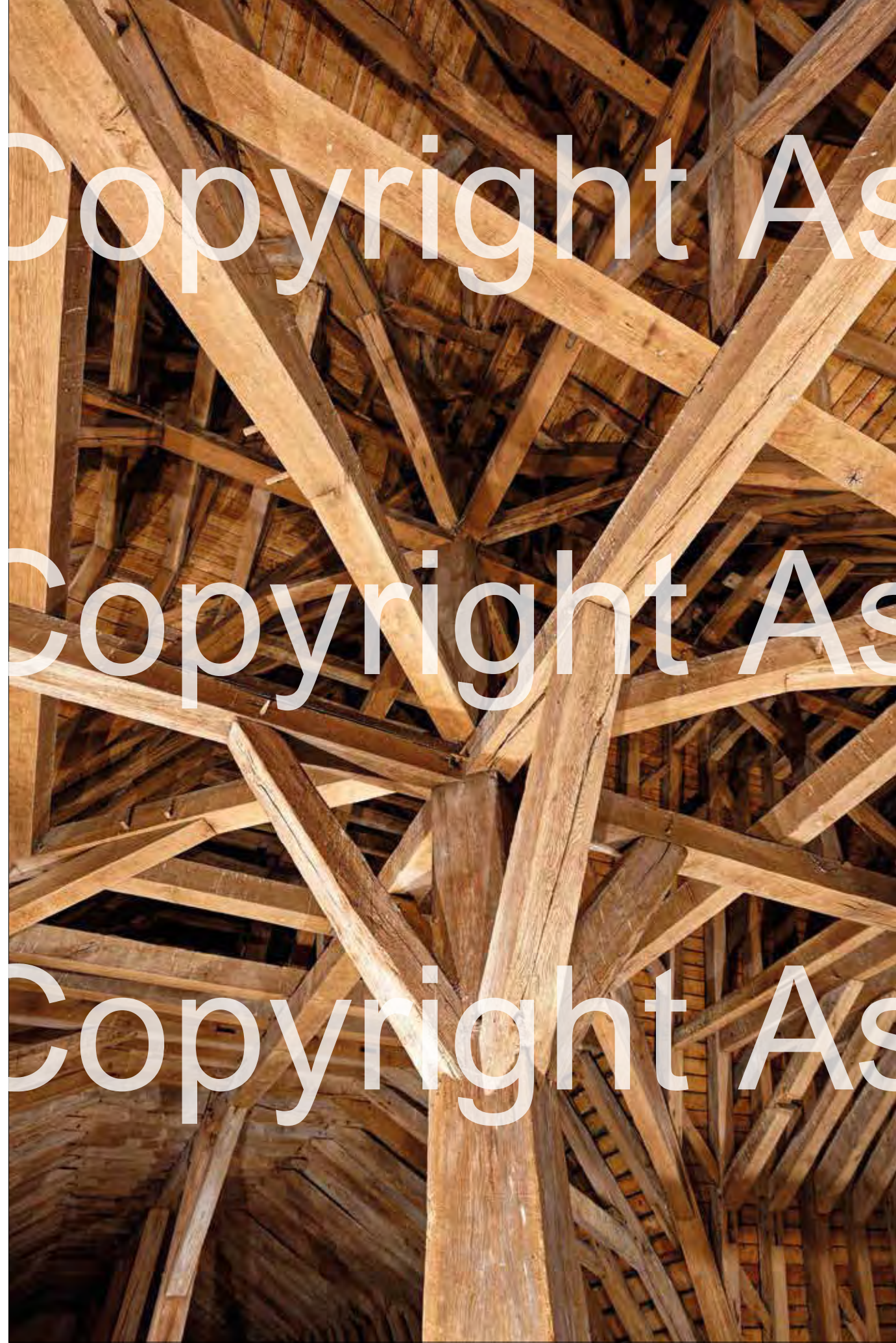
A single post on two large intersecting tie-beams supports the trusses at the junction of the nave and transept roofs.
