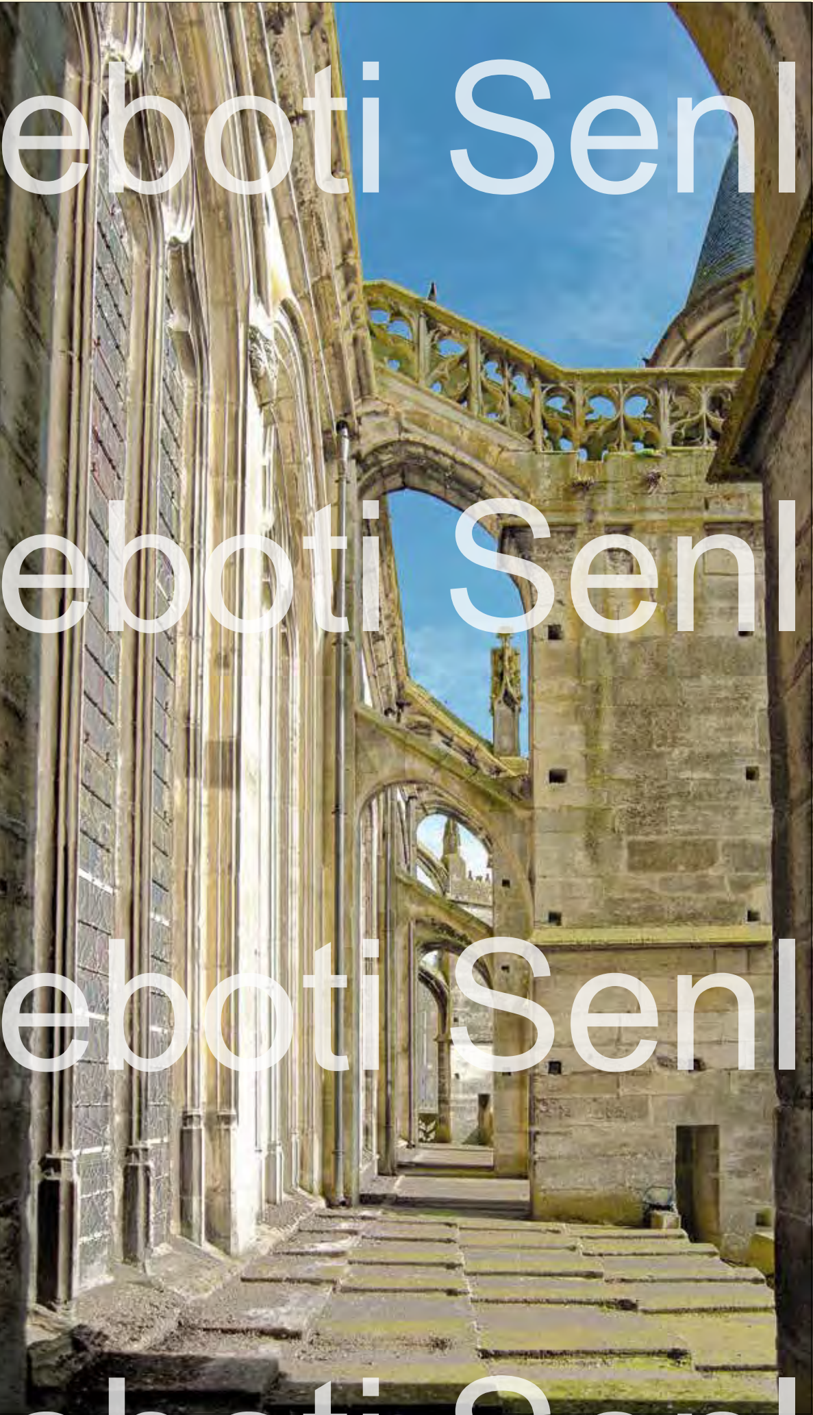
Flying buttresses above the south side chapels.
