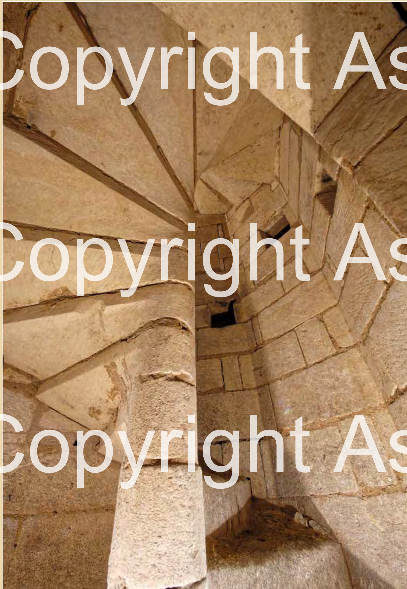
An octagonal stone spiral staircase with a solid stone central shaft. Possibly dating from the 15th century, this staircase is constructed as a turret within the cellar, rather than being embedded within the walls.
