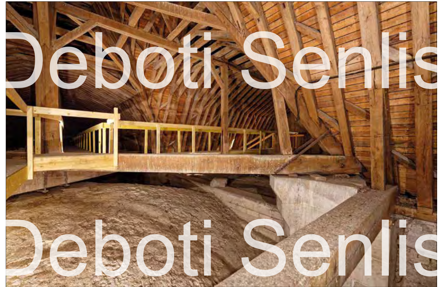
The wooden roof structure does not rest on the vaults.
